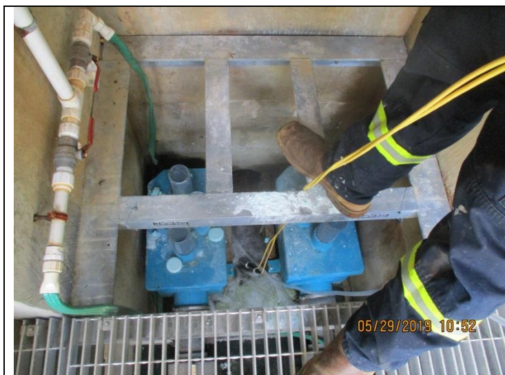
7. Close-up view of dechlorination tablet feeders.
