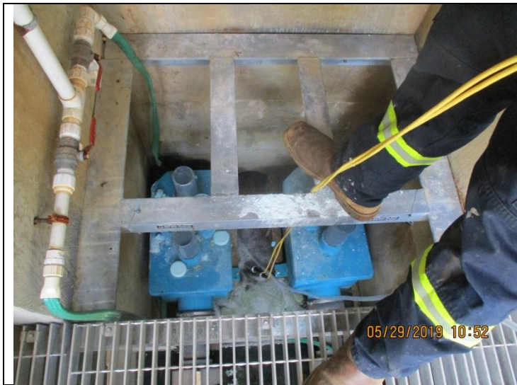
7. Close-up view of dechlorination tablet feeders.
